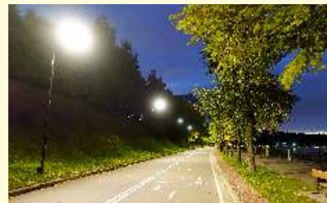
Street Lights Lining the Roads
